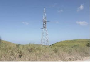
Plate 6 - 132 kV Transmission Line Towers 28m high
