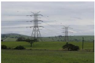
Plate 5 - 400 kV Double Circuit
