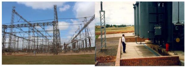
Plate 1 - Sub-station Busbars maximum height 22.5m
