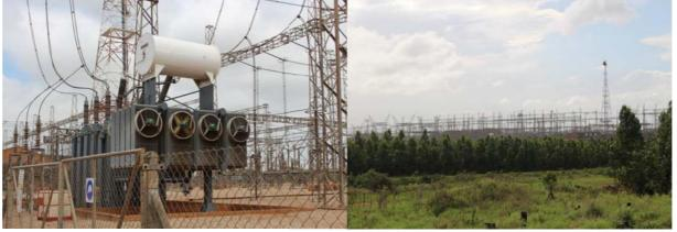
Plate 3 - Transformer showing oil reservoir and fans for cooling
